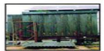
OIL & GAS PCR (POWER CONTROL ROOM)
